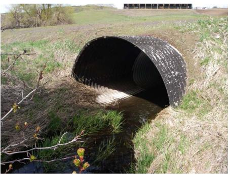
Photo 8: Airport Creek crosses Airport Road via this squashed CMP. The cross-section of this CMP measures to be 7 feet in height and 11 feet in width.
